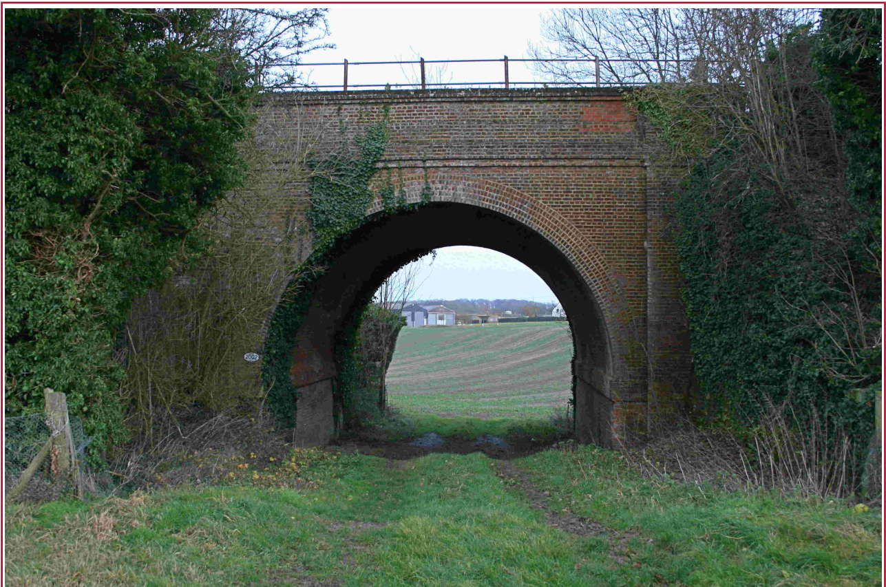
Illustration v: Railway bridge at B from north
