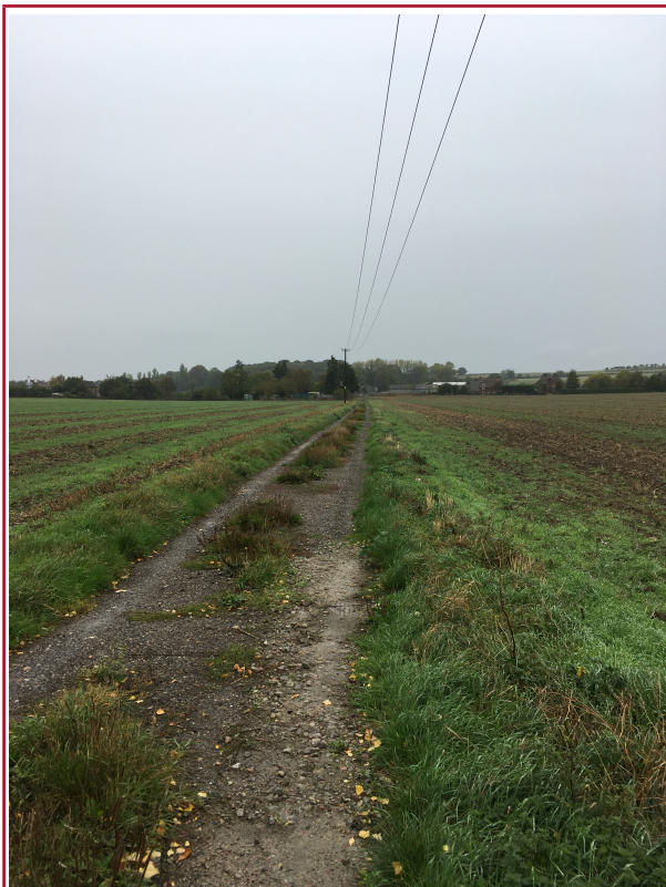
Illustration iv: Second pumping station towards A
